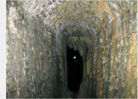
8. One of the underground tunnels.
